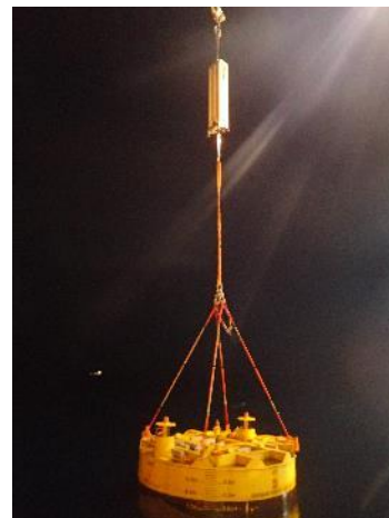
Figure 10-2 Dynamic Model for lifting in air with PHC (left), Photo of PHC during installation (Courtesy: Safelink)
