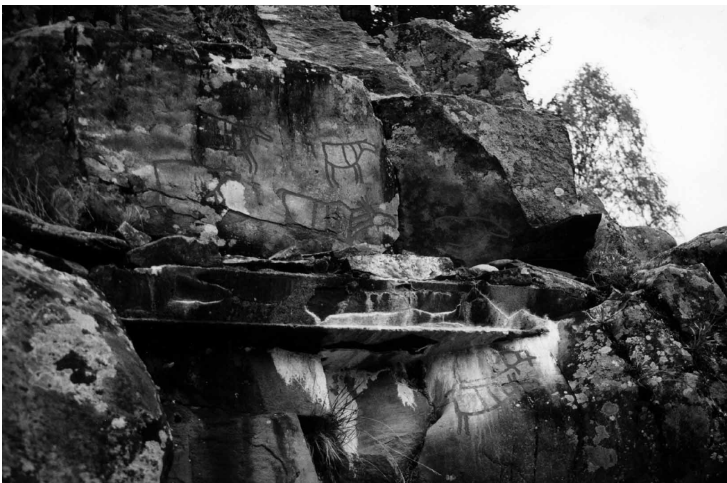
Fig. 6. The rock art site Drotten, Fåberg, Gudbrandsdalen in year 2000. Calcium from the level concrete bar, and from concrete fill in cracks above, has leached and then re-deposited as calcite on the rock and partly on some of the carvings. The result at Fåberg is an unexpected and ugly curatorial mistake, but can this process under controlled conditions be used for strengthening heavily weathered rock art panels? Photo: I. M. Olsrud.
