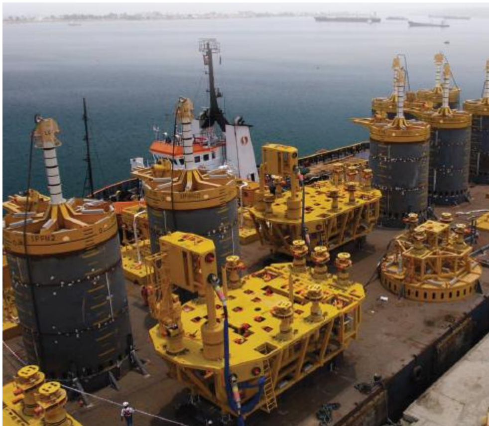
Figure 33 Typical subsea manifolds set up for installation in offshore (GE oil and gas, 2011)
