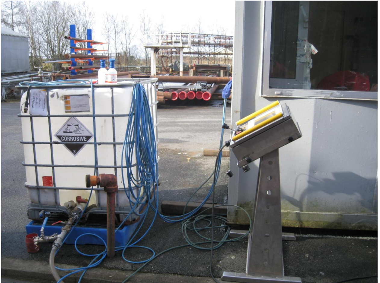
Appendix 16: HT- 400 control panel
