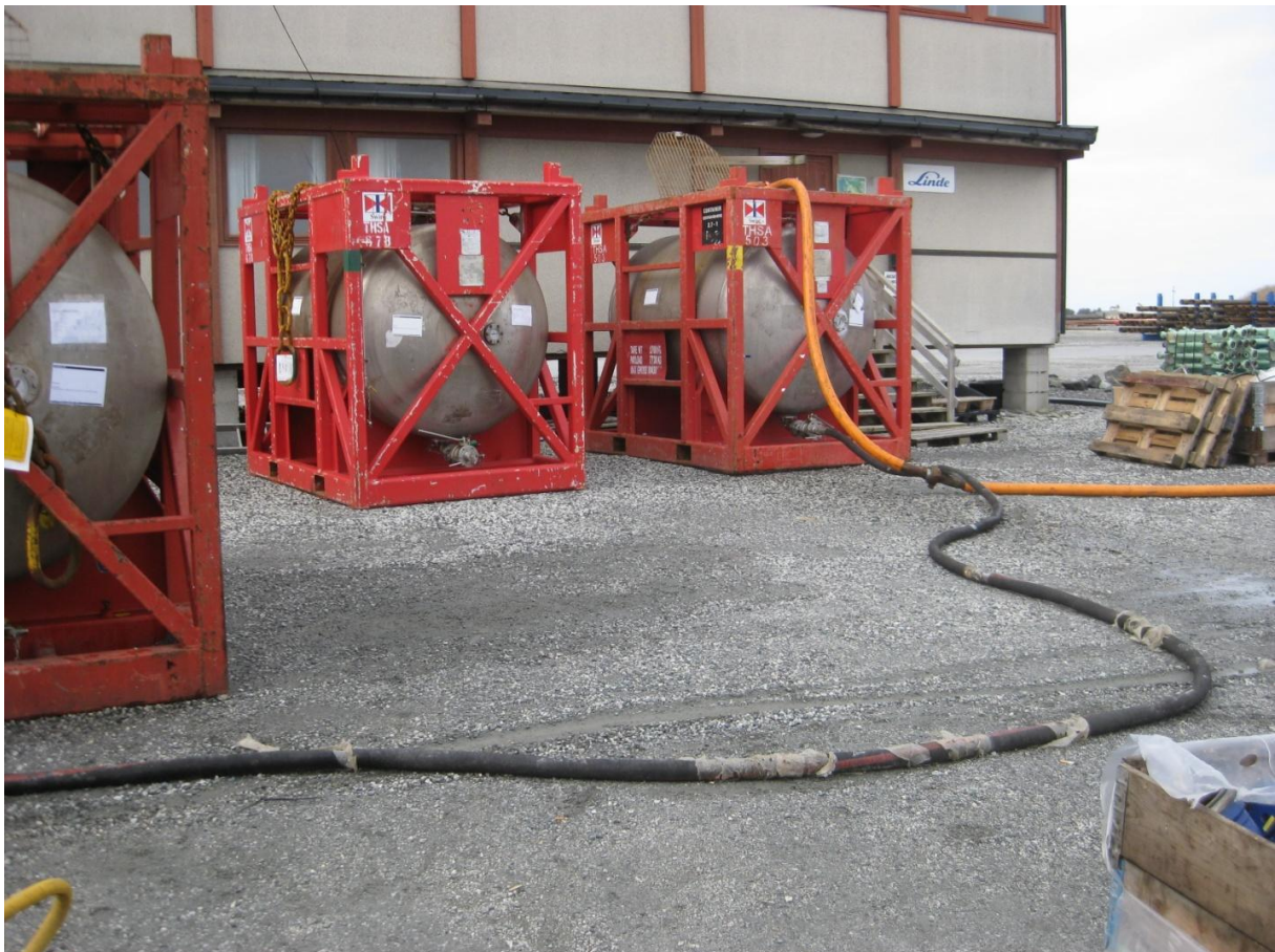
Appendix 4: Gel tank and water tank at test site
