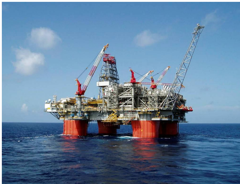
Figure 23 Picture of Thunder Horse production and drilling platform in the Gulf of Mexico. ©GVA
