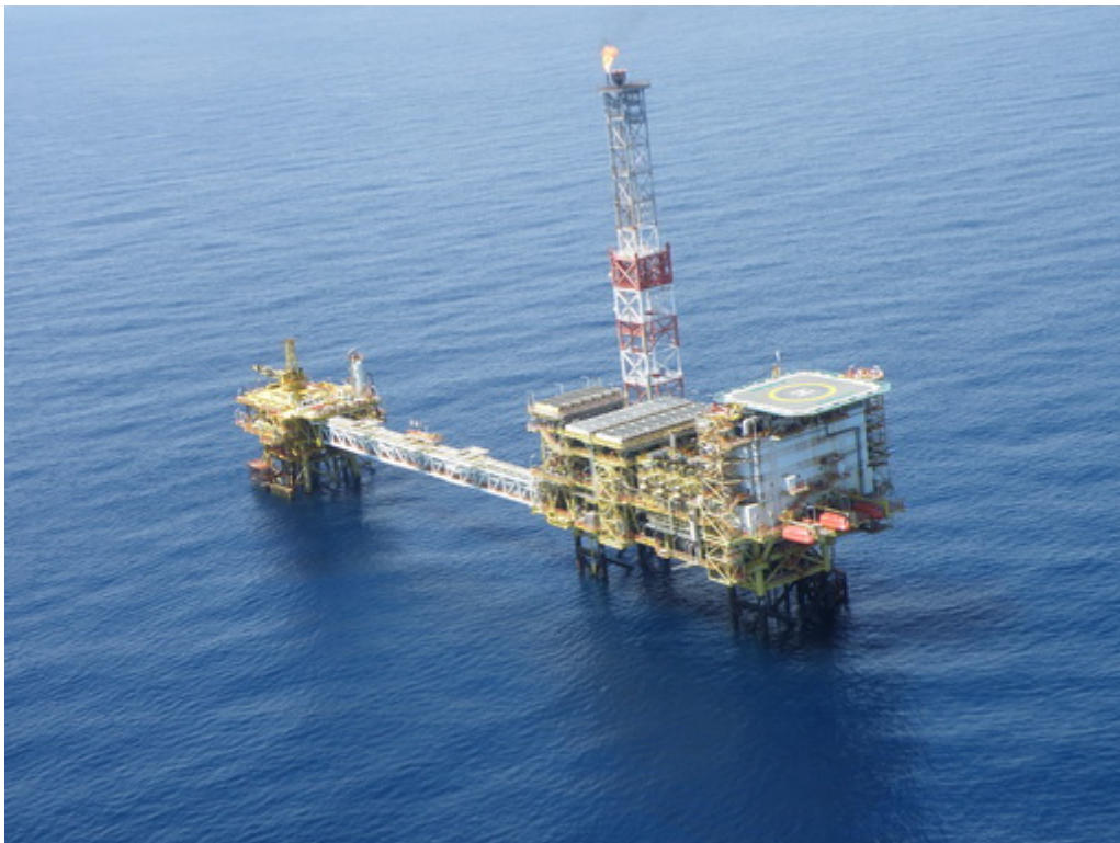
Figure 1: an offshore helideck (Helideckinspect, 2013)
