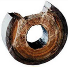
Figure 4-22- Scale in production tubing [45]
