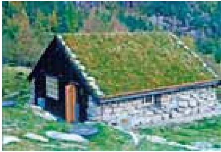
Fig. 1.3.7. RBC housing solution. BK NuDisc installed at a Youth Hostel in Norway to treat wastewater to a high degree including nutrient removal. During winter this 150 pe plant treats wastewater from Caretaker's of 4 persons only, but in summer the population can increase to 150 persons and for a short period of 4 or 5 weeks the population peaks to about 200 persons. The plant is installed in a building due to the extreme cold weather in Norway. (From www.keeprocess.com )
