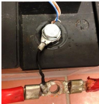
Figure 6.12: Specially designed fuse.
