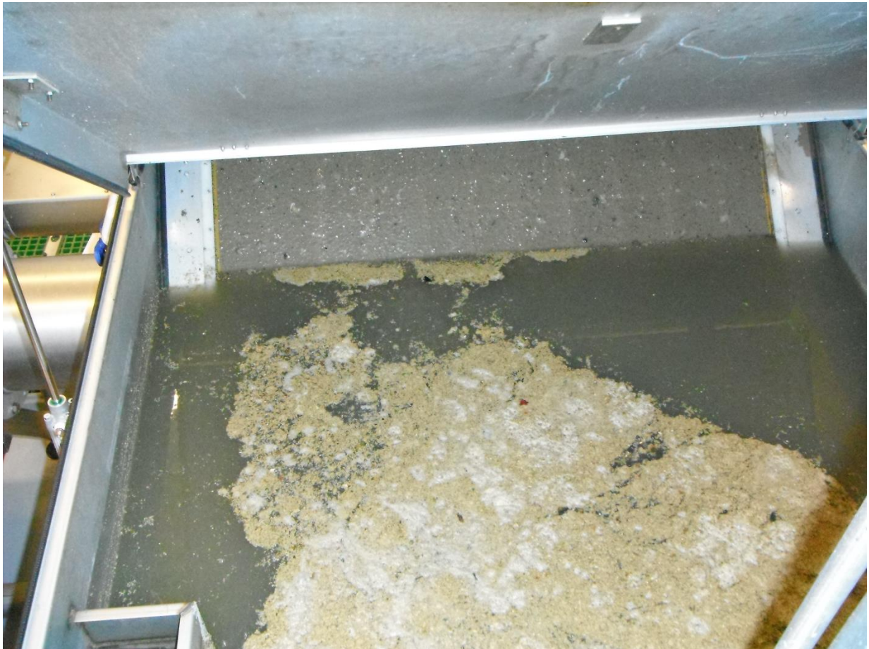
Figure 50: Fats floating in SF6000 prior to filter in Tiendeholmen Renseanlegg in Namsos.
