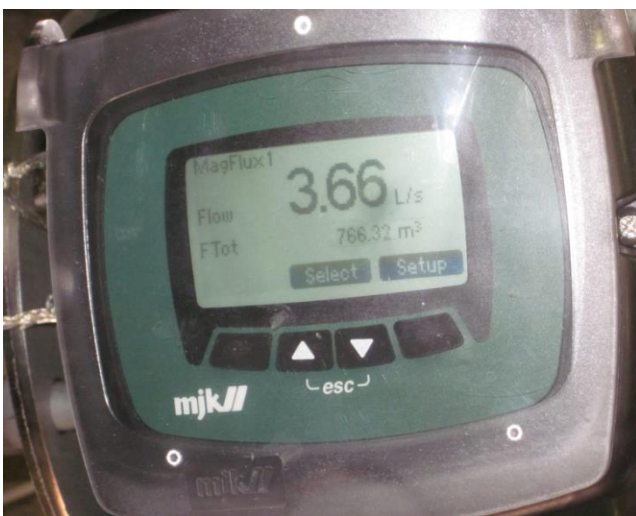
Figure 15: attached magnetic flux flow meter
