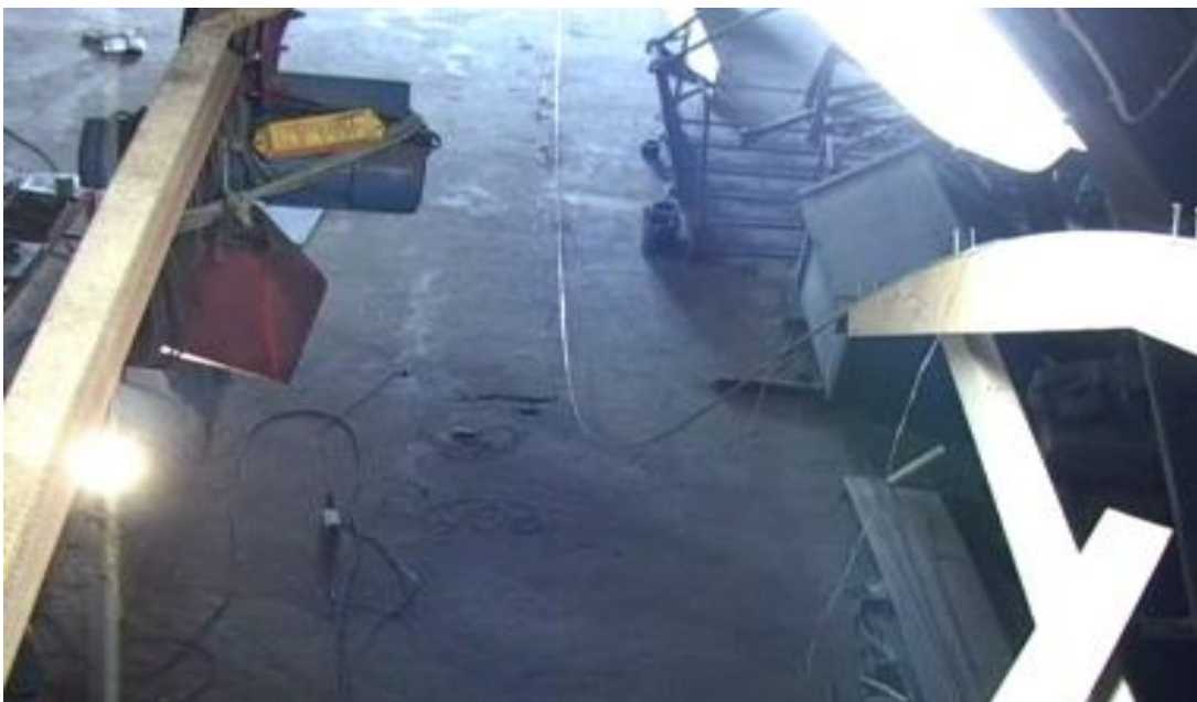
Figure 10d. Pipeline laid from 4.97 meters height
