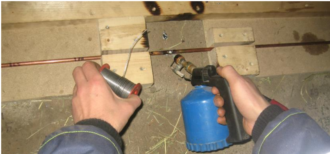
Figure 12. Soldering of the joints
