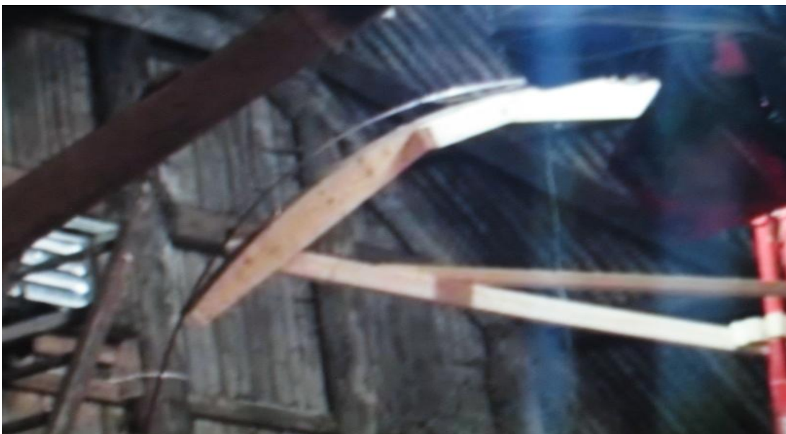
Figure 74. The stinger as the lift was moved.
