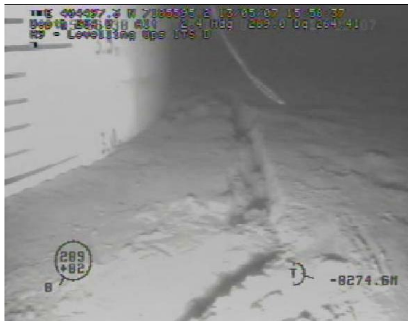
Figure 5.1: Wash out during installation [15]
