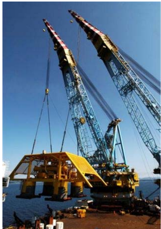
Figure 3.6: Lift of Tordis SSBI with use of Saipem 7000 [1]
