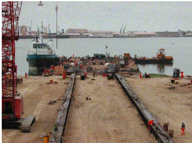
Figure 3.4: Skidding ways in yard [1]
