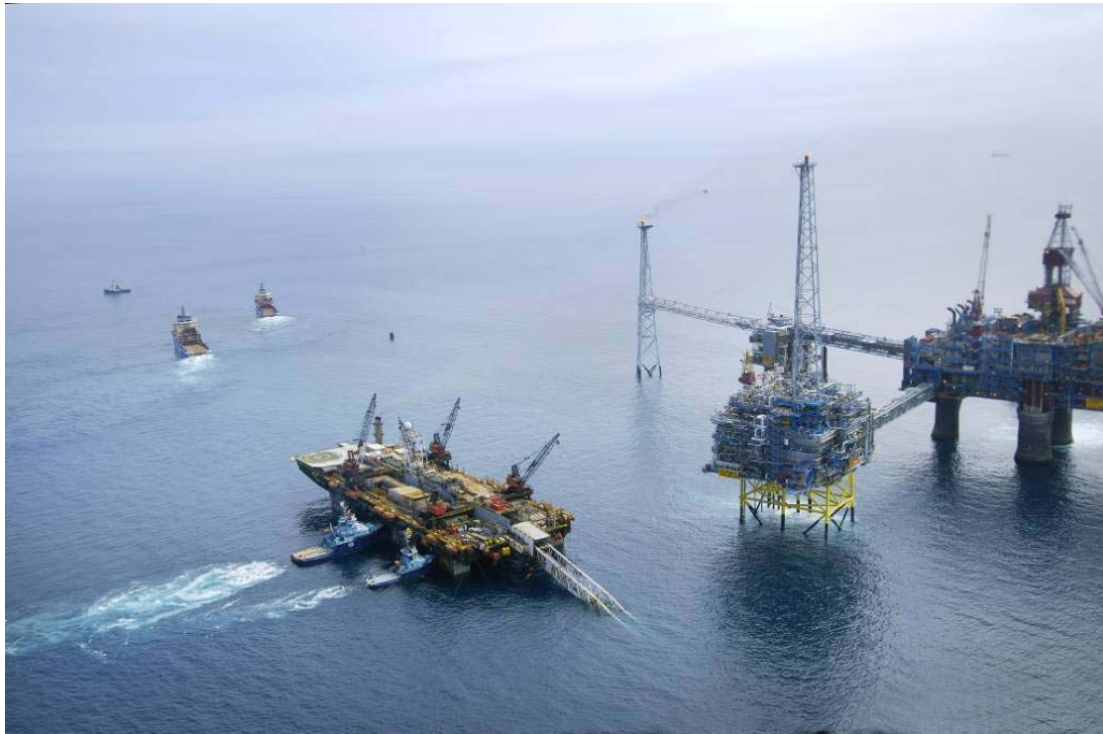
Figure 1.1: Picture shows Acergy Piper during pipe lay close to Sleipner field centre. Several marine operations are in action; pipe lay, anchor handling, extra pushing tugs, pipe supply vessel (outside picture) and a survey vessel to monitor touchdown (outside picture). [1]
