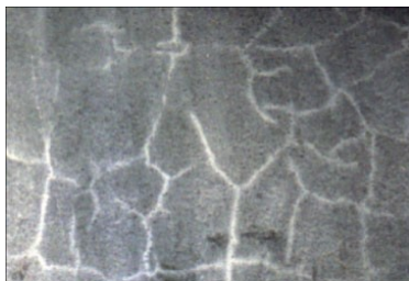
Figure 2-5: Plastic shrinkage,ref[12]
