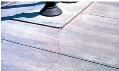
Figure 2-8: Drying shrinkage ref[15]
