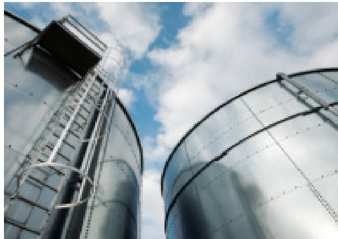
Figure 14: Gravity separator tanks [26]
