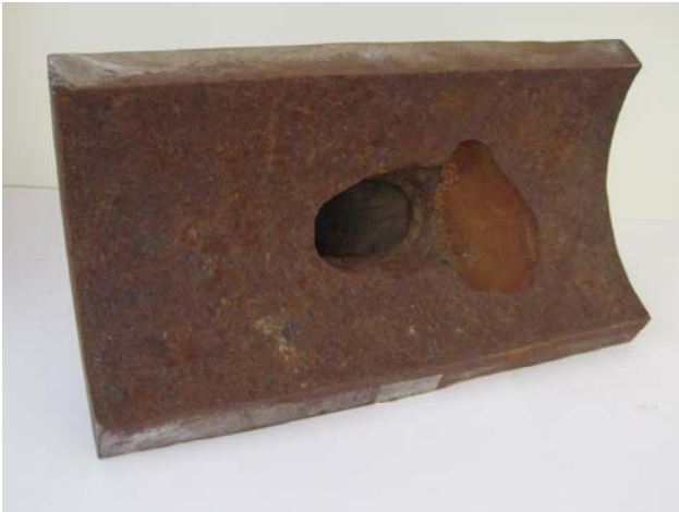
Figure 2.8: Corrosion due to presence of chemicals and turbulence and welded wall
