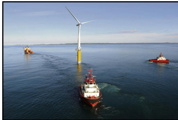
Illustration 10 The Hywind 1 floating turbine is towed to its test site off Karmøy, Norway. Photograph: Statoil
