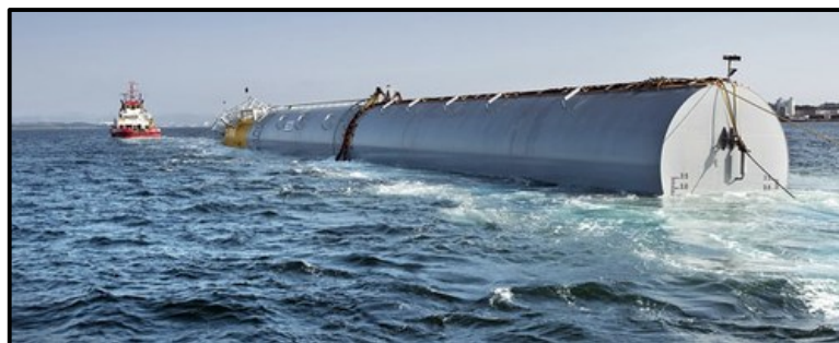
Illustration 11 Hywind tow floating windmill at sea in deep water (Photo: Kim Laland/StatoilHydro)
