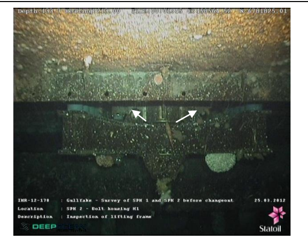
Figure 4.25: Lifting Frame and secure pins
