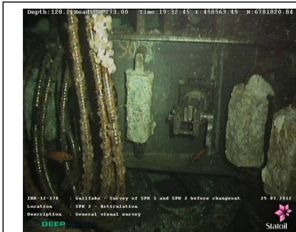
Figure 4.39: Access to H2 Safety Locking Pin
