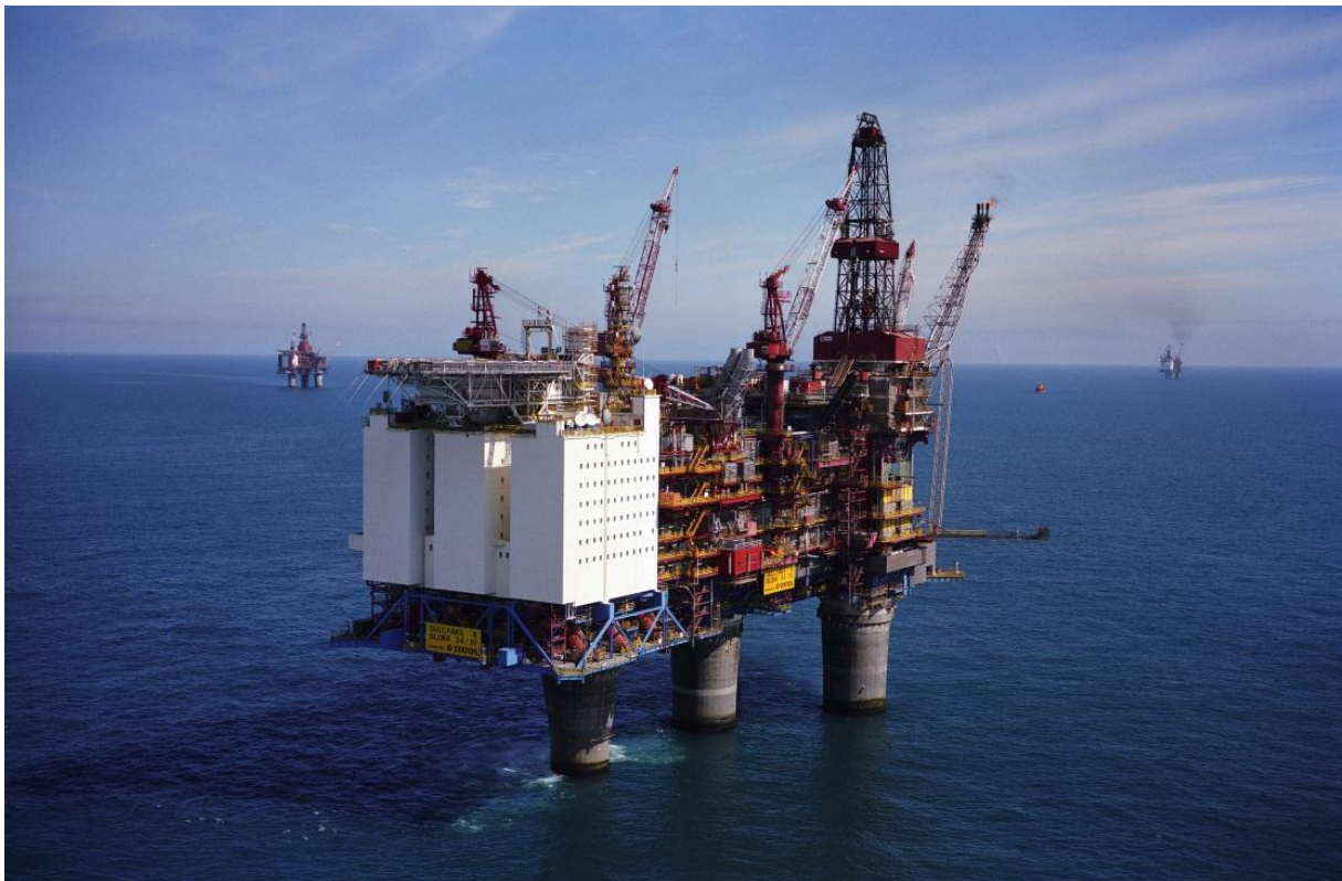
Figure 2.5: The three Gullfaks coondeep platforms[20]
