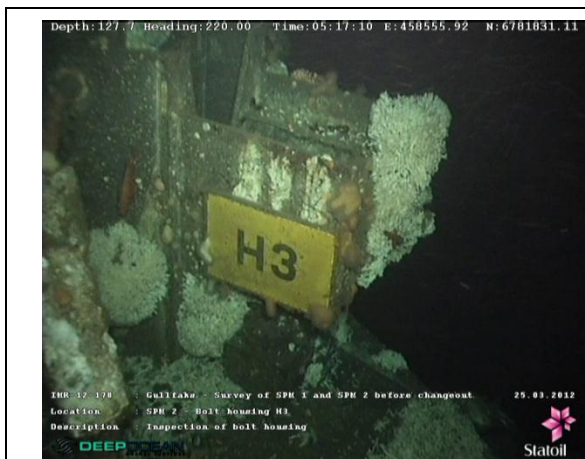
Fig 4.18: Side of bolt housing H3
