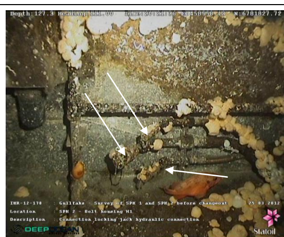
Figure 4.36: Locking Bolt Quck Couplings
