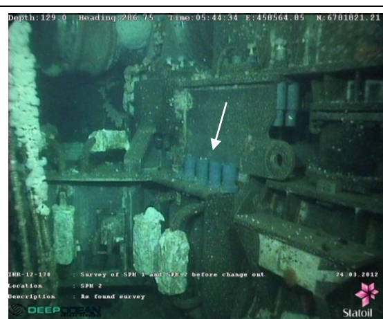
Figure 4.23: Foundation bolts, south side
