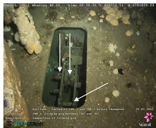
Figure 4.38: Safety pin and safety spike
