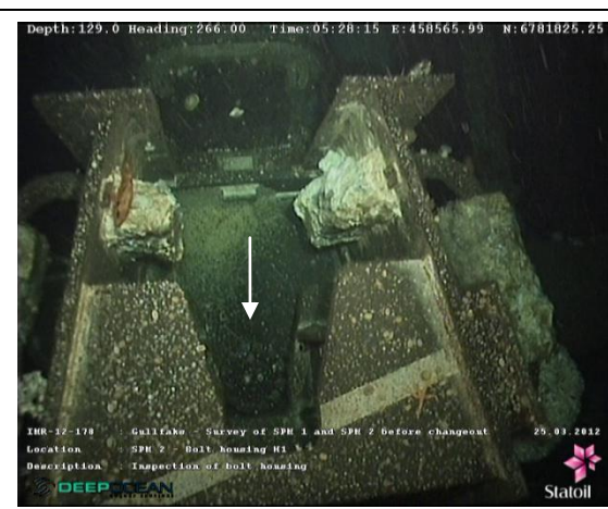
Figure 4.9: Behind bolt housing with flange
