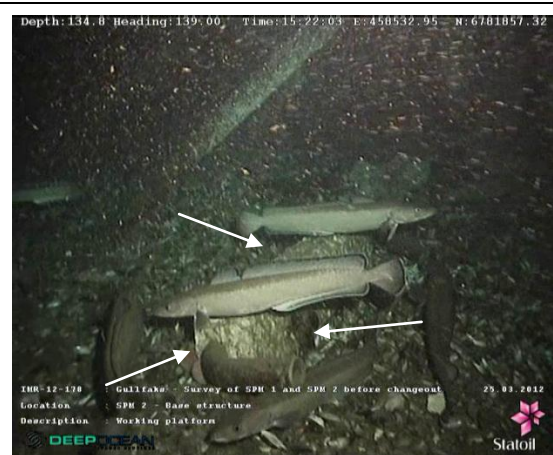
Figure 4.7: Loose anode on working platform
