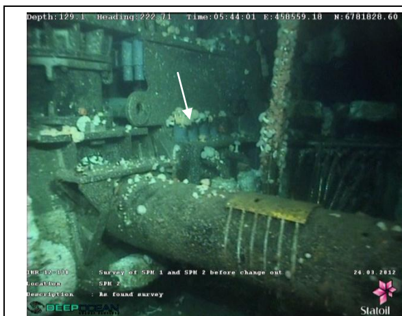
Figure 4.22: Foundation bolts, north side
