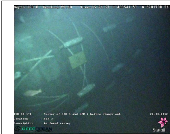
Fig 4.6: Pontoon with stand-off anodes
