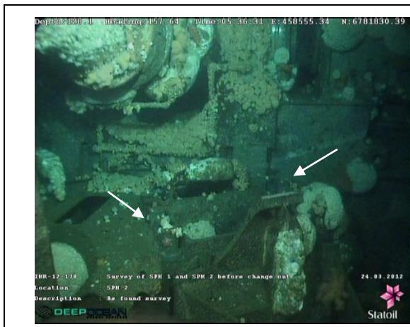
Figure 4.30: Foundation Bolts North-East Side
