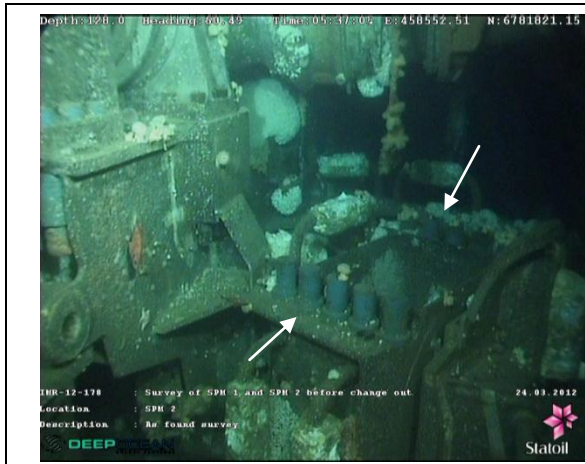
Figure 4.26: Foundation Bolts North-West Side
