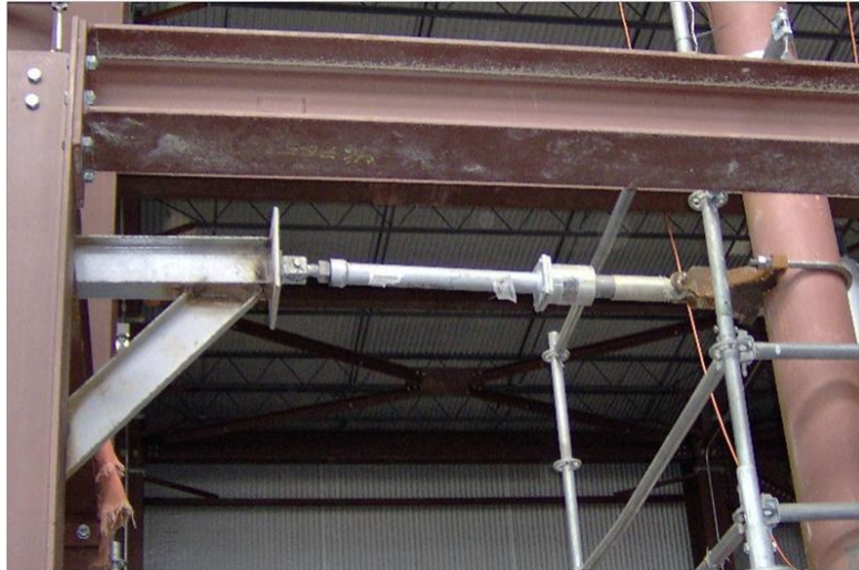
Figure 19. Mechanical snubber on site (Wikipedia, 2011)
