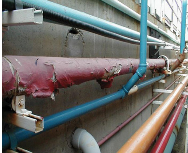
Figure 6. Improper choice of jacketing (Lettich, 2007).
