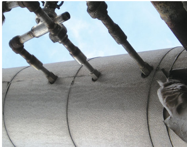
Figure 10. Sealant problems of jacketing (Lettich, 2007).
