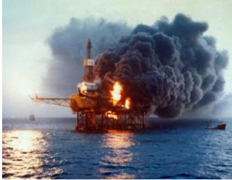
Figure 6 : Destroyed Piper Alpha oil rig in North sea
