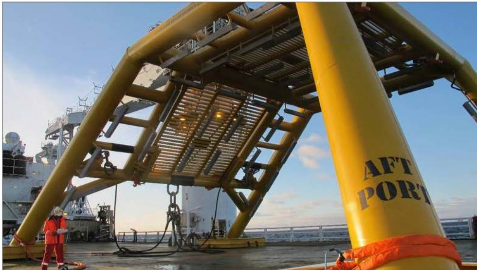
The recent underwater Asgard field operation took place from subsea contractor Technip's "Skandi Arctic" vessel. FOTO: Technip
