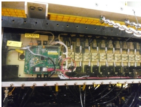
Figure 9-31 SCM 01 valve pack
