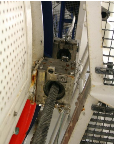
Figur 7 Guide wire leading up to the winch
