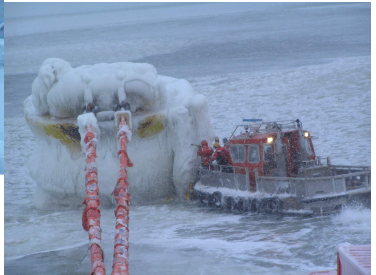
Figure B-4. Icing on SALM (Single Anchor Leg Mooring) on Sakhalin II. (Canatec Associates International Ltd, 2004)
