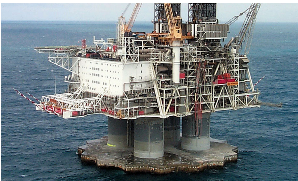
Figure 12. Hibernia Platform off the Coast of St John's, New Foundland (Hibernia, 1997)
