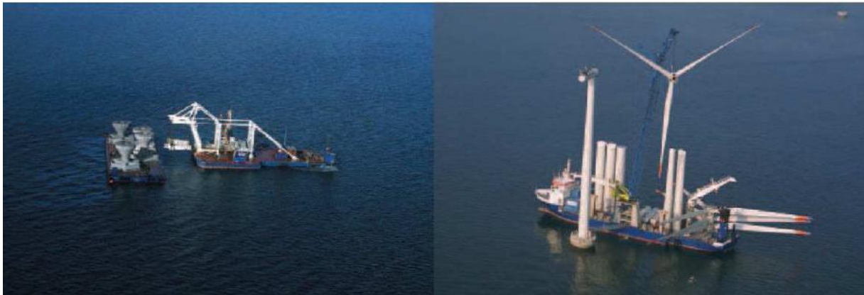
Image 1: To the right; barge type installation of an offshore wind turbine. To the right; ship based installation of an offshore wind turbine [15].
