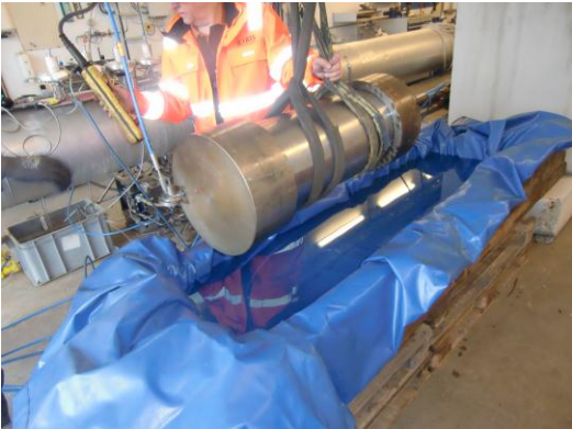
Figure 6-11: Installing Test Equipment for Alt. 1 for Pressure Test at IRIS
