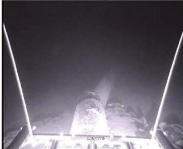
Figure 3-6 Kvitebjørn pipeline showing displacement caused by anchor (Gjertveit, et al., 2010)
