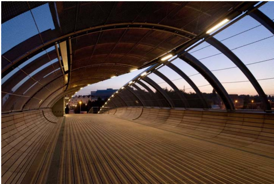
Figur 78. Villetaneuse footbridge i Frankrike. Foto: Cyril Sancereau, Jean-Paul Houdry
