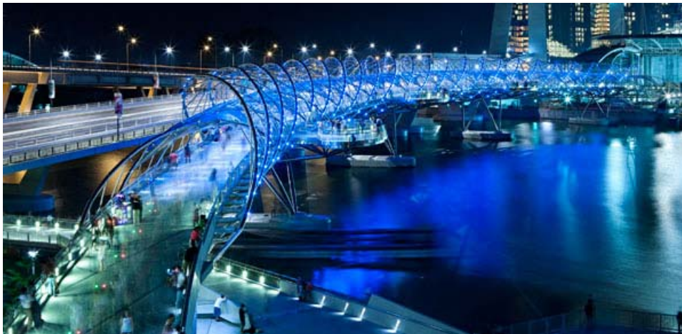
Figur 76 Cox-Rayner Helix Bridge. Kilde: http://www.evolo.us/architecture/
