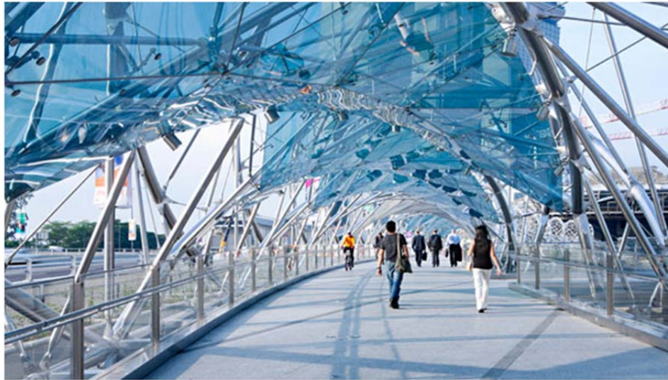
Figur 75 Cox-Rayner Helix Bridge. Kilde: http://www.evolo.us/architecture/
