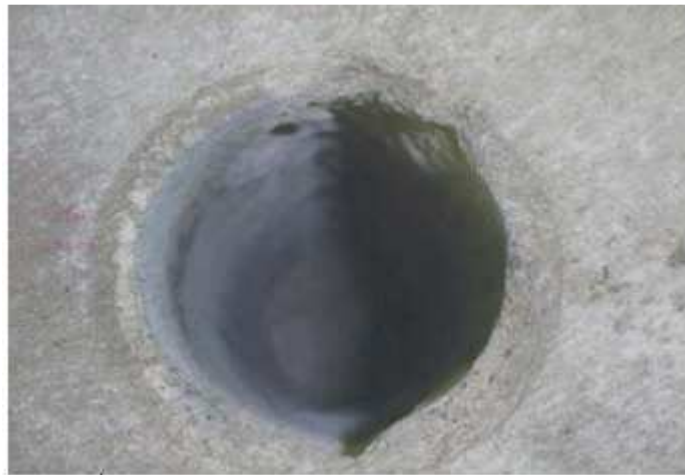
Figur 1-4 Borehole Breakout due to a directional
