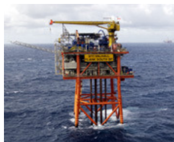
Figure 2.1.3: One of the flank platforms at the Valhall field. [BP, 2009 f]
