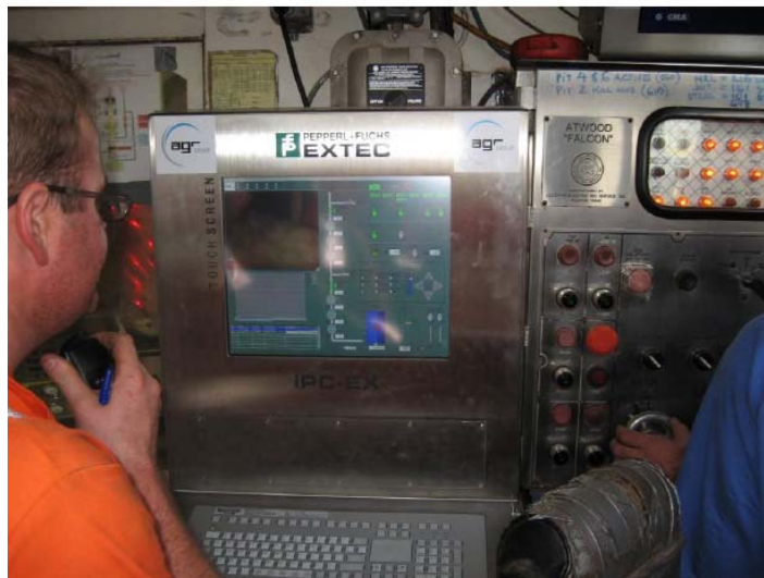
Figure 35: RMR control panel in driller's cabin 13
