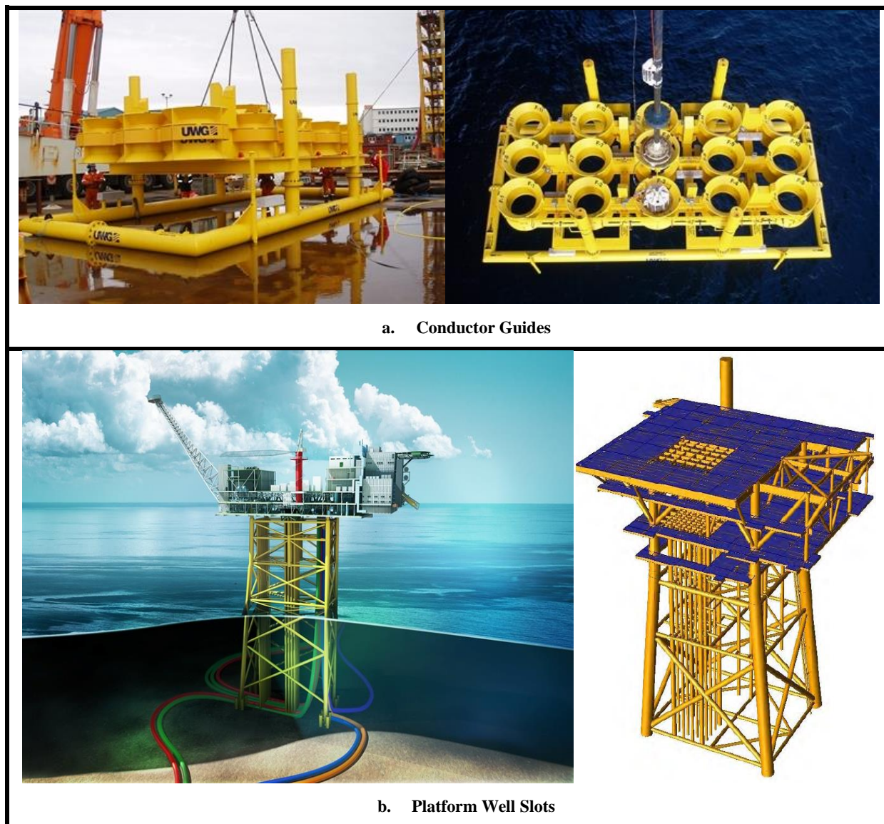
Fig. 5.12. Conductor Guides and Platform Slots [26].
