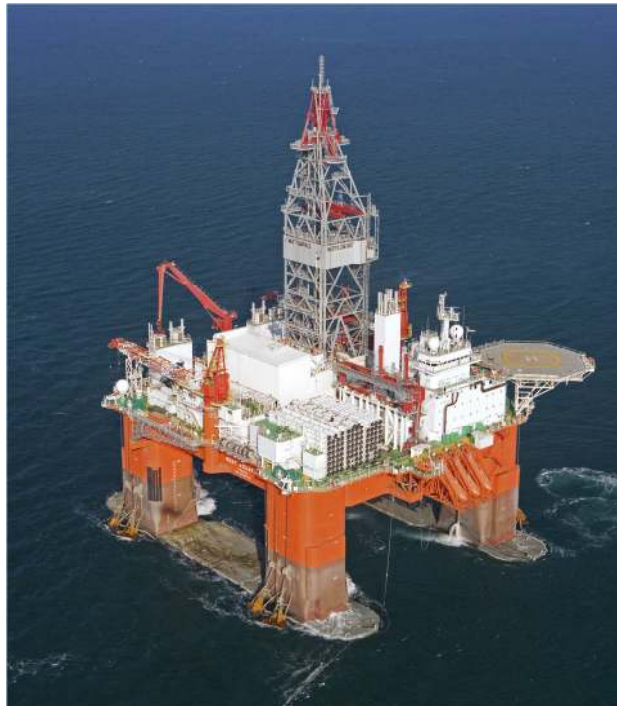
Figure 10 - West Aquarius, a semi-submersible with derrick tower [25]
