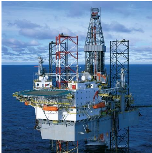
Figure 1 Drilling with jack-up at the Aries field by Offshore technology.com
