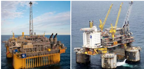
Figure 4: Two semisubmersible production units, Troll B with both production and drilling facilities and Troll C with production facilities, also used for producing the Fram field. [23]
