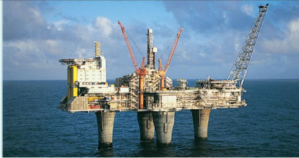
Figure 3: Purpose built concrete platform, Troll A, attached to seabed. [23]
