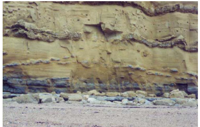
Figure 14: Calcite-cemented concretions and developing layer. [7]
