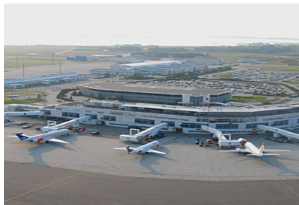
Photo 2. Overview of Stavanger airport. Note. From Ramboll, "Stavanger Lufthavn, Sola" by Nyhus, (n.d.). Copyright n.d. by Ramboll.
