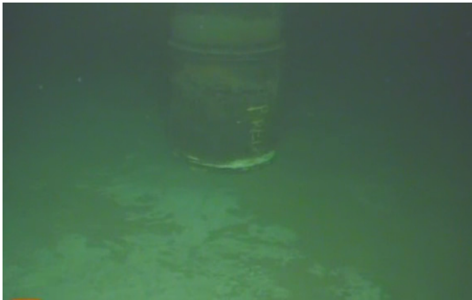
Figure 39 Conductor after grouting cement job [71]
