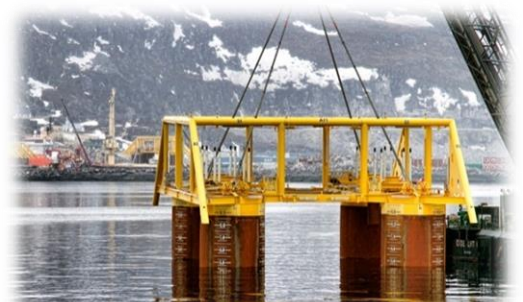
Figure 29. Subsea unit installation [eninorge.com]
