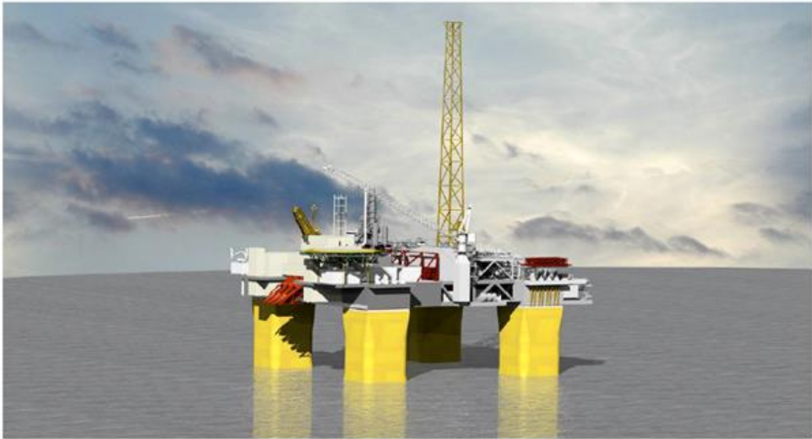
Figure 5: Picture of the platform, a semi-submersible floating platform. (PUD plan, internal GDF SUEZ document)
