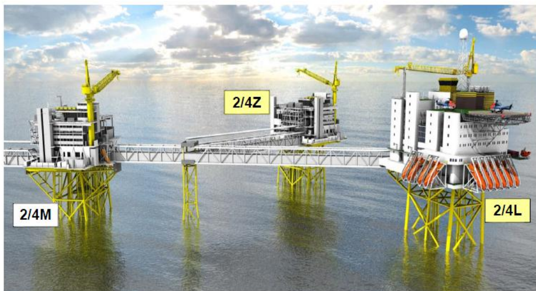
Figure 2.1: Placement of the new 2/4 L platform.
