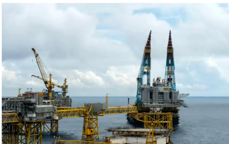
Figure 2.6: Installation of living quarter 2/4L on the Ekofisk field.
