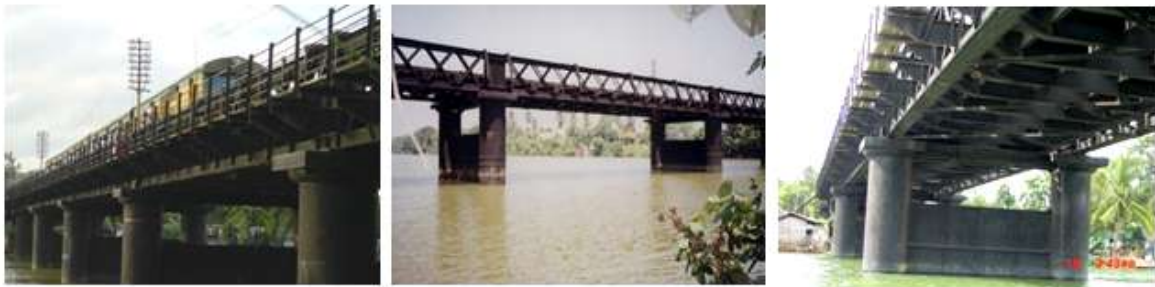
Figure 39 General view of the riveted railway bridge [30]
