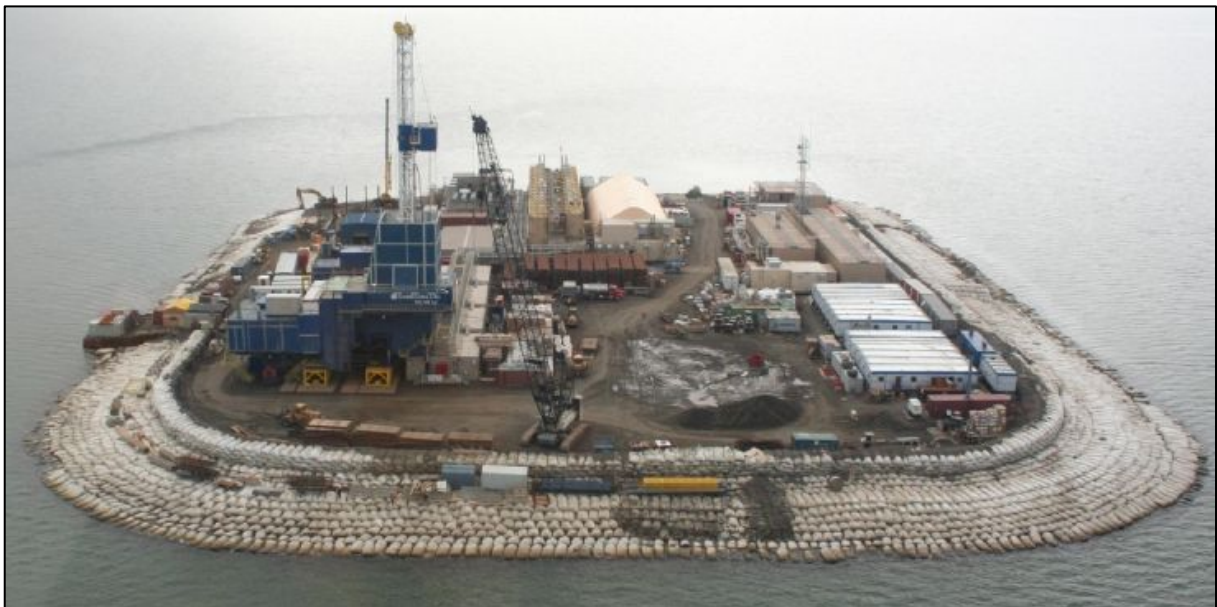
FIGURE 4.11 OOOGURUK ARTIFICIAL DRILLING AND PRODUCTION ISLAND [77].
