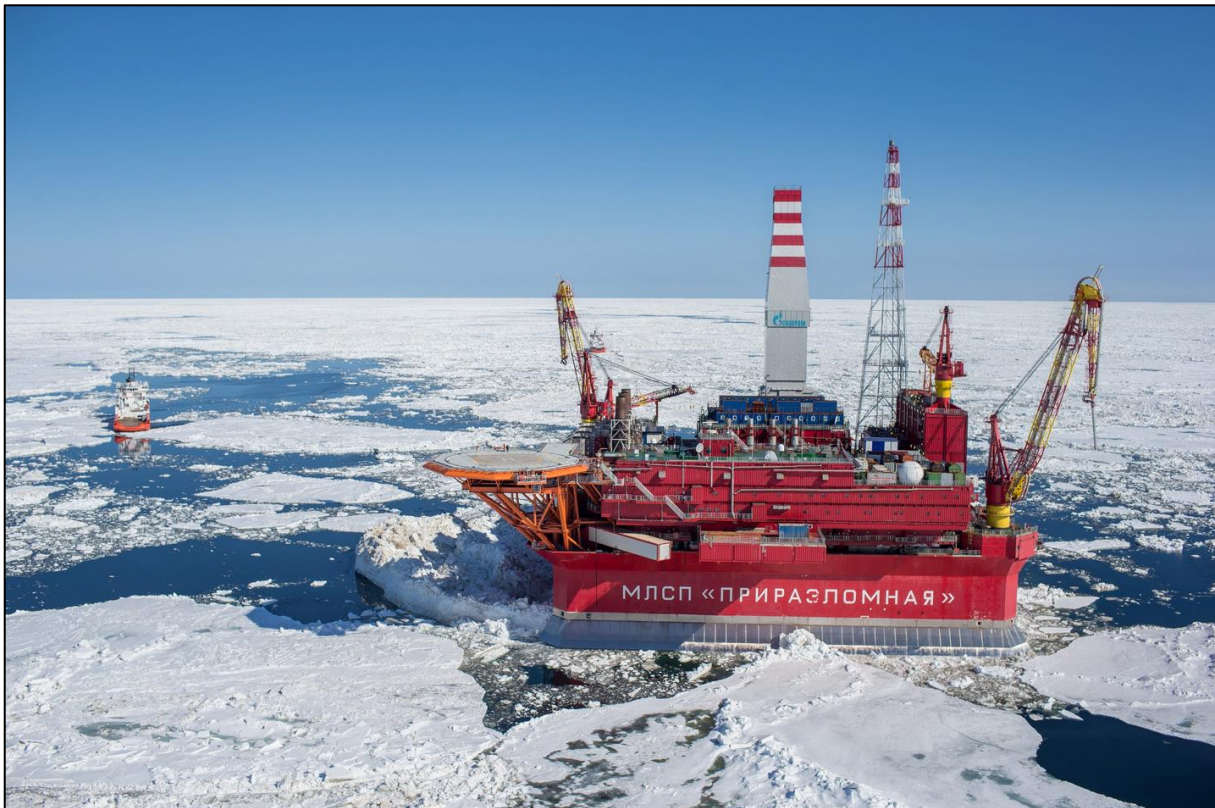
FIGURE 4.12 PRIRAZLOMNOYE DRILLING AND PRODUCTION CAISSON [78]
