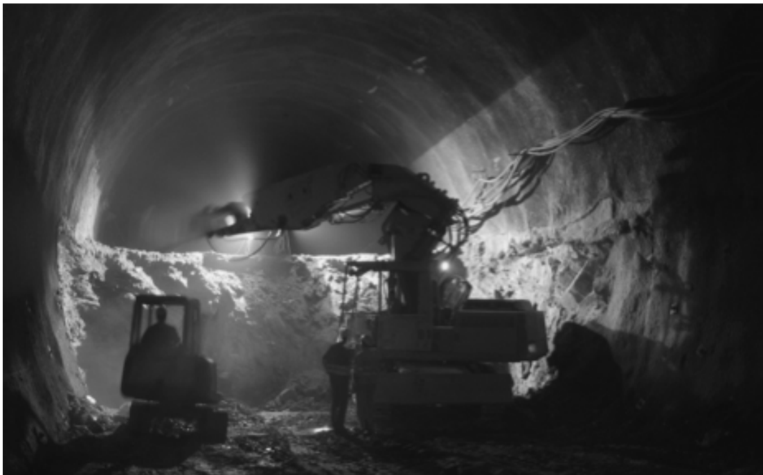
Figure 3-6 Example of using an excavator during a NATM
