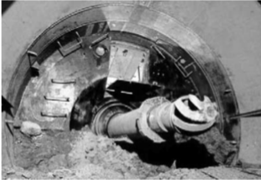
Figure 3-12 Thixshield excavation header, used for selective excavation
