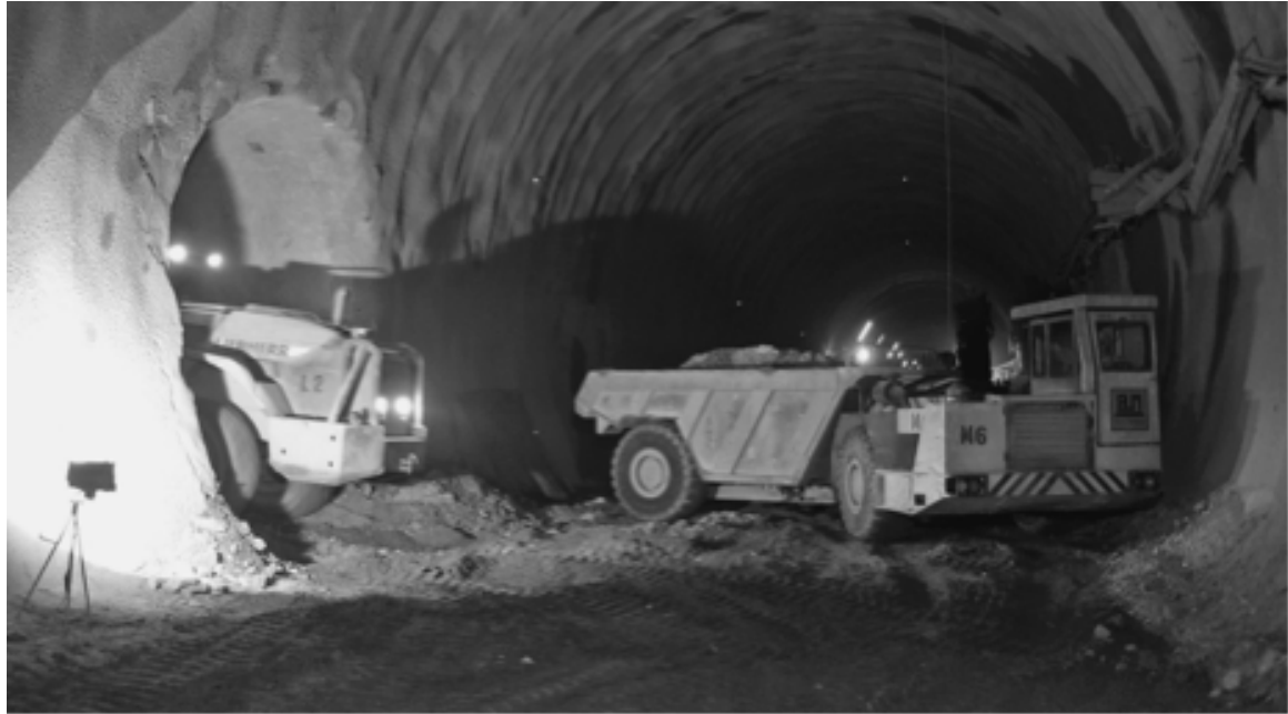
Figure 3-1 Example of an emergency cross passage under construction
