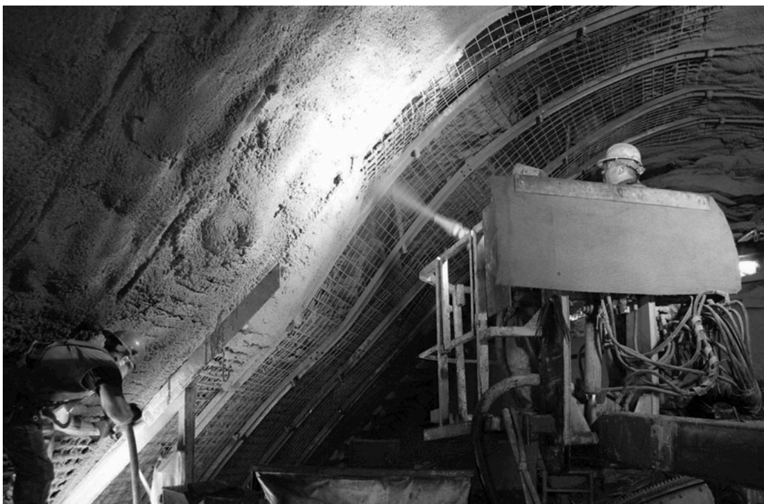
Figure 3-7 Example of shotcreting mesh reinforcement
