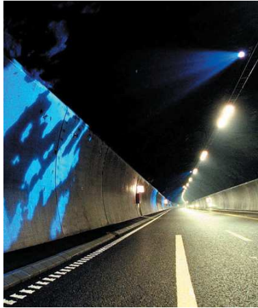
Figure B.2: Artistic light patterns are projected onto the tunnel wall in order to break monotony of the tunnel (Melby et al., 2002).
