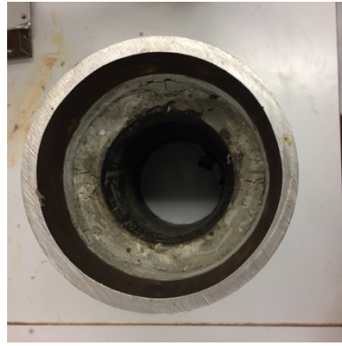
Figure 45: D Tube number 4 with 1,8 cm cement thickness.
