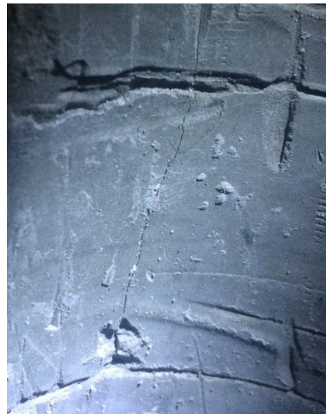
Figure 69: Test result from setup 2. Minor damage to the cement and fractured to the top of cement.
