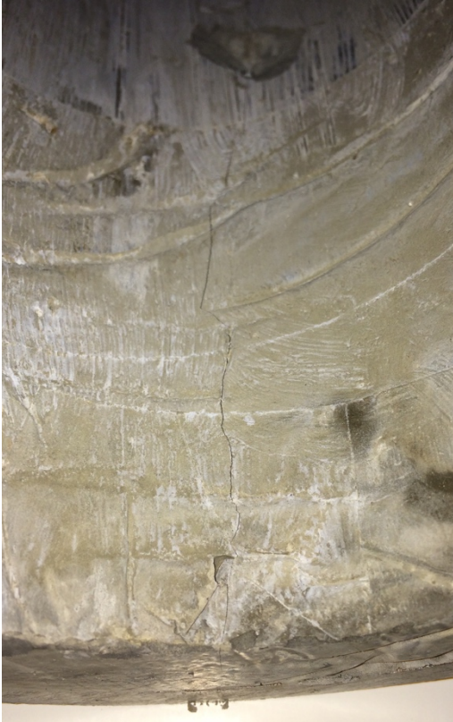
Figure 56: Test result no. 4: The crack has propagated down to the bottom of the tube. The picture is taken from bottom of the tube.
