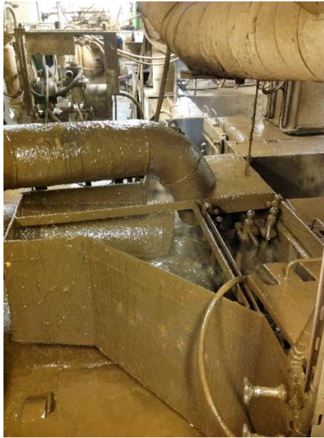
Figure 18: Header box geometry on the right side of the flowline outlet at the semi-submersible drilling rig.
