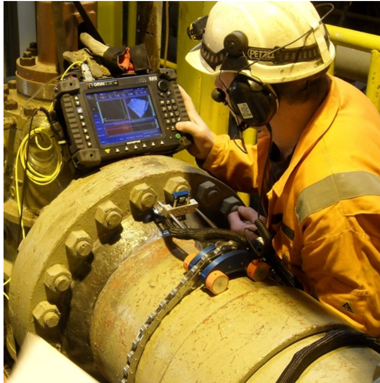
Figure 32 - Phased Array Testing on Pipe Spool (Courtesy of Aker Solutions MMO)
