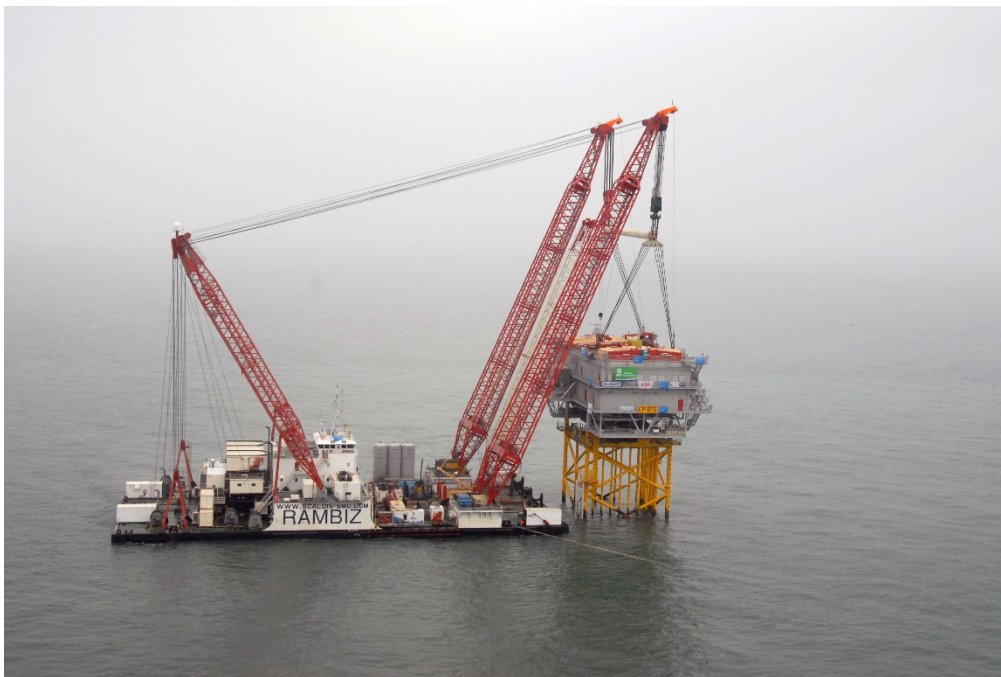
Figure 5-1 Installation operation. Taken from web link: www02.abb.com
