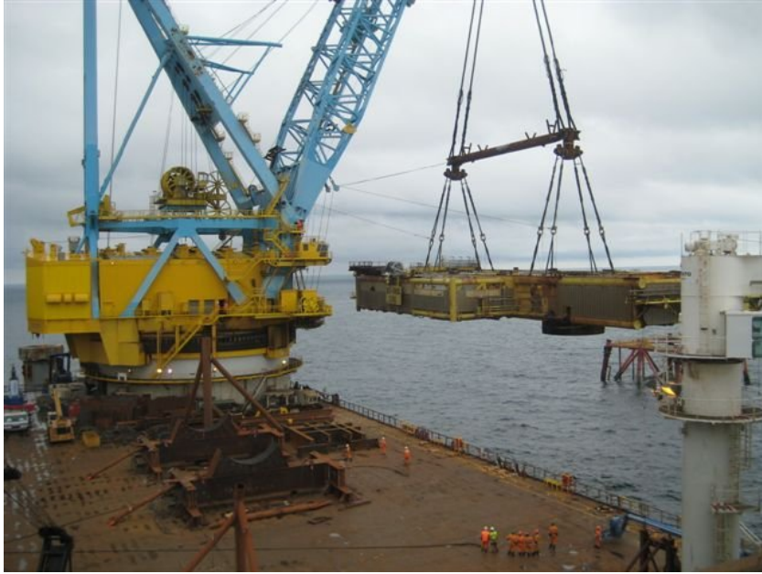
Figure 4-4 Lifting using spreader bars. Taken from web link: www.hollandiaoffshore.nl
