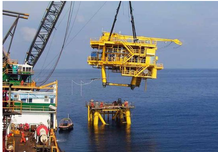
Figure 4-1 Typical offshore lifting. Taken from web link: http://www.chain-connection.com
