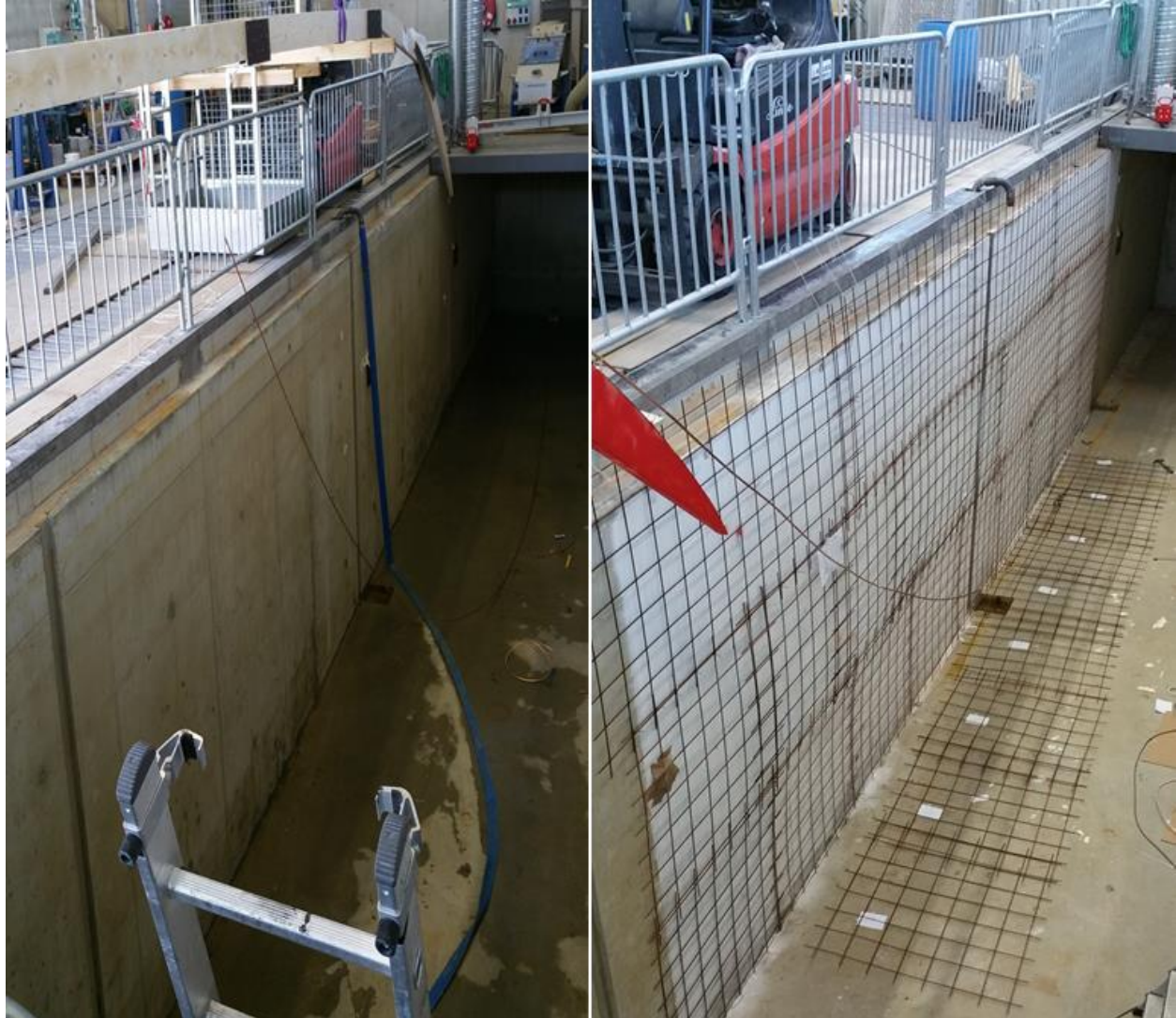
Figure 5-6 Pool wall preparation. Before and After preparation for experiment tests.
