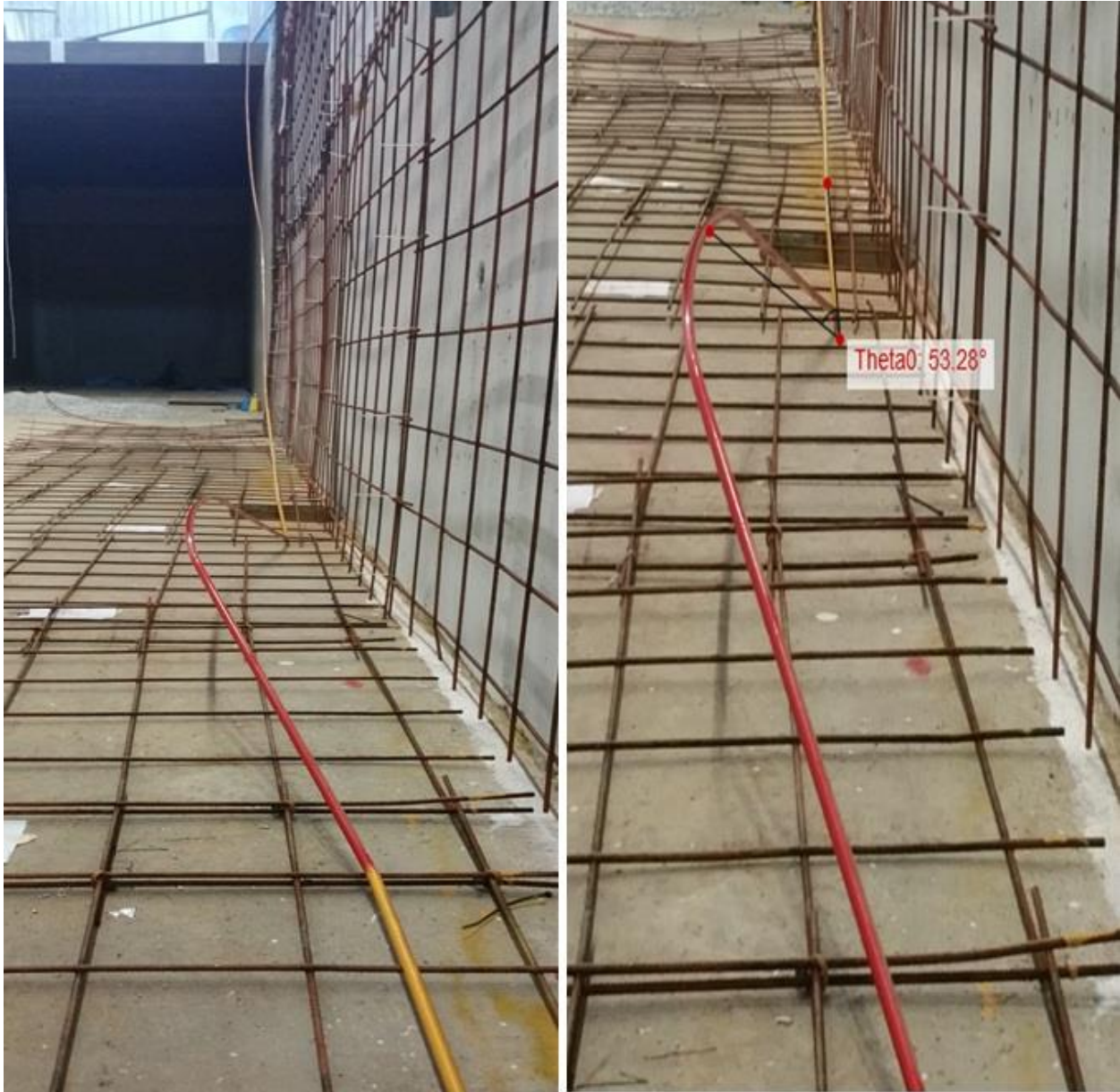
Figure F5- for test 8, See Section 7.3.8 for installation parameters.
