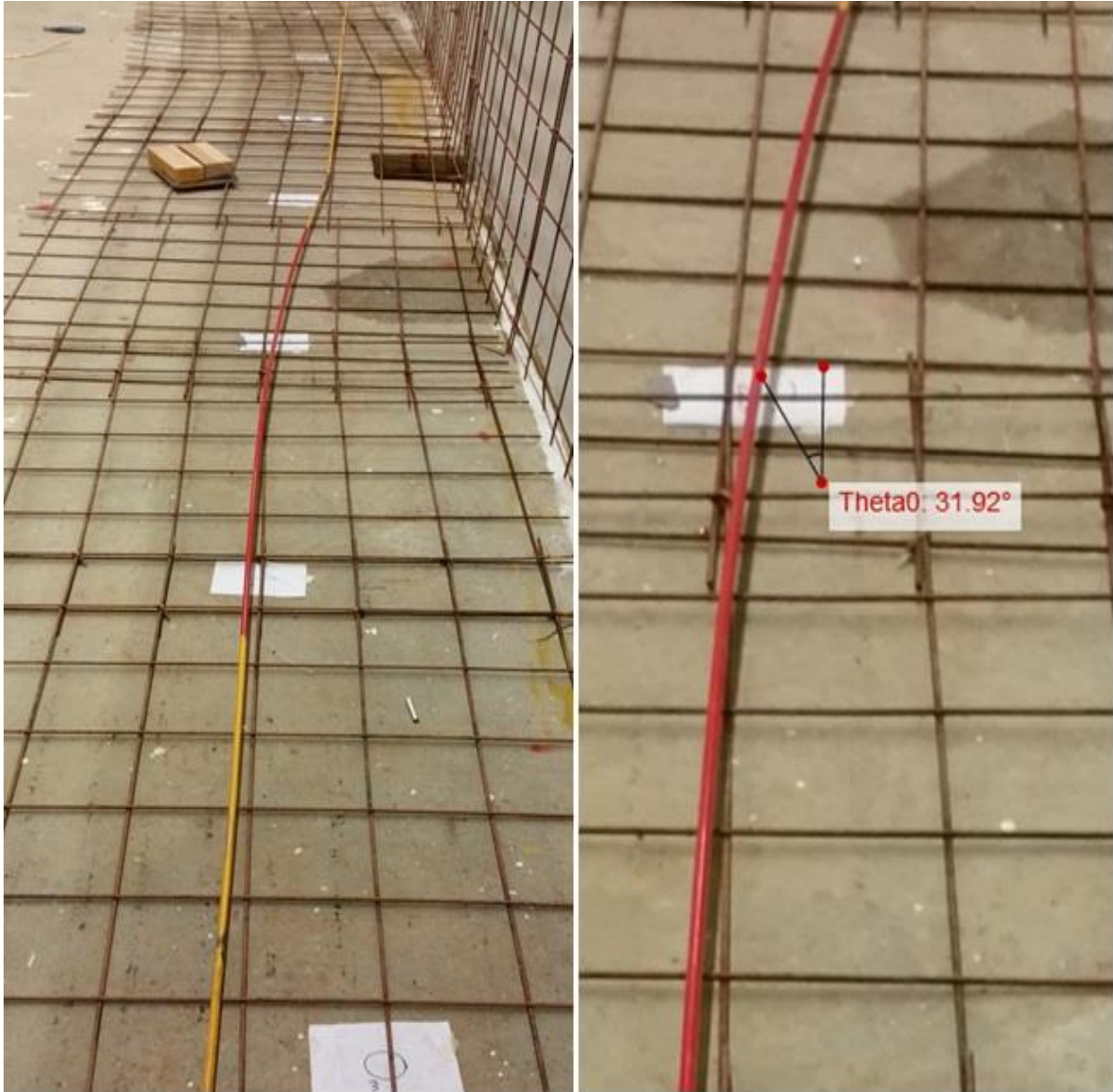
Figure F3- for test 5, See Section 7.3.5 for installation parameters.
