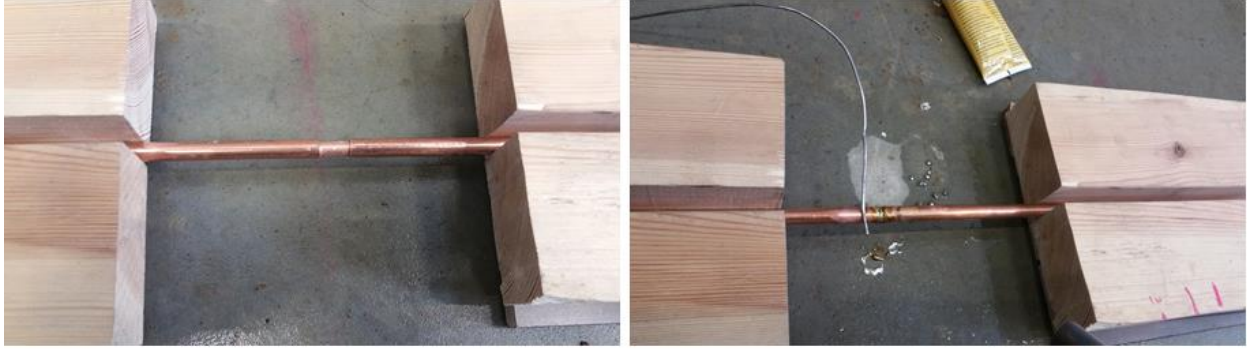
Figure 5-4 Soldering of pipes, Small diameter pipe is used inside at connections
