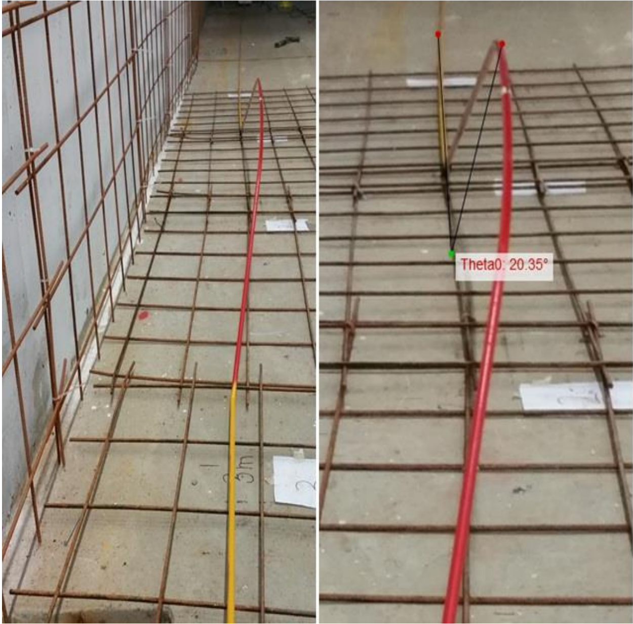
Figure F8- for test 13, See Section 7.4.3 for installation parameters.
