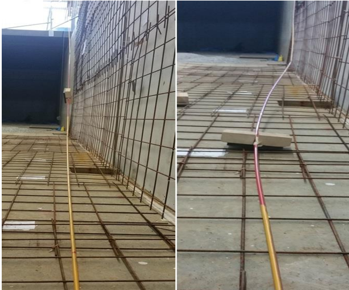
Figure 7-10 Test 7: Left side: start of the experiment. Right Side picture: Pipe is at TDP, pipe and inline structure rotated 90 degrees.
