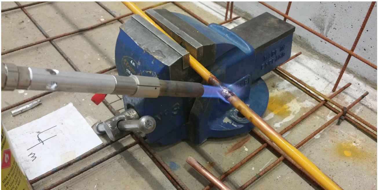
Figure 5-5 Heating of pipe joint for disconnecting the pipe
