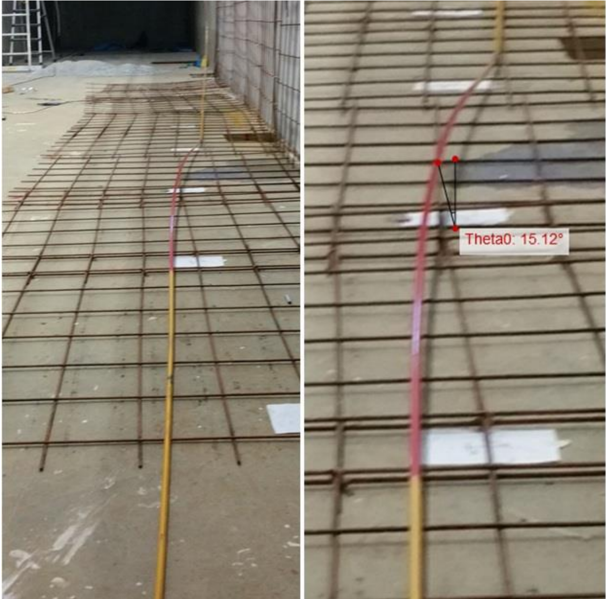
Figure F2- for test 4, See Section 7.3.4 for installation parameters.
