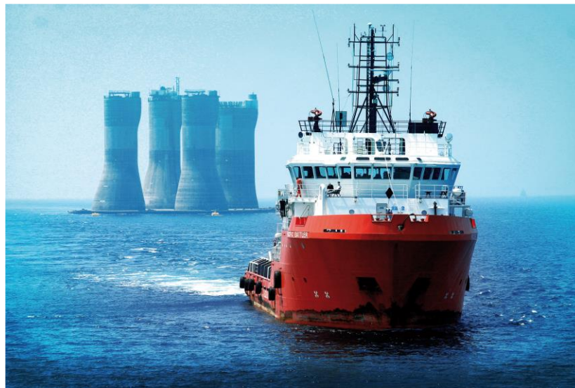
Figure 47. Towing of one of the Sakhalin II concrete GBSs from Vosthosny Port to field location outside Sakhalin Island
