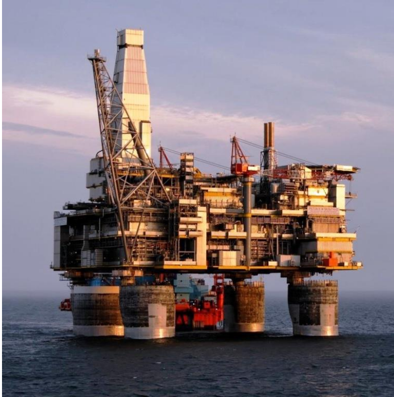
Figure 17. Piltun-Astokhskoye-B (PA-B) platform (Photo courtesy of Sakhalin Energy Investment Company).
