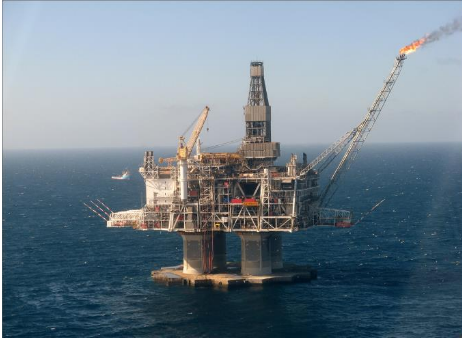
Figure 43. Hibernia platform with multi-shaft GBS (Photo courtesy of Hibernia Management and Development Company)
