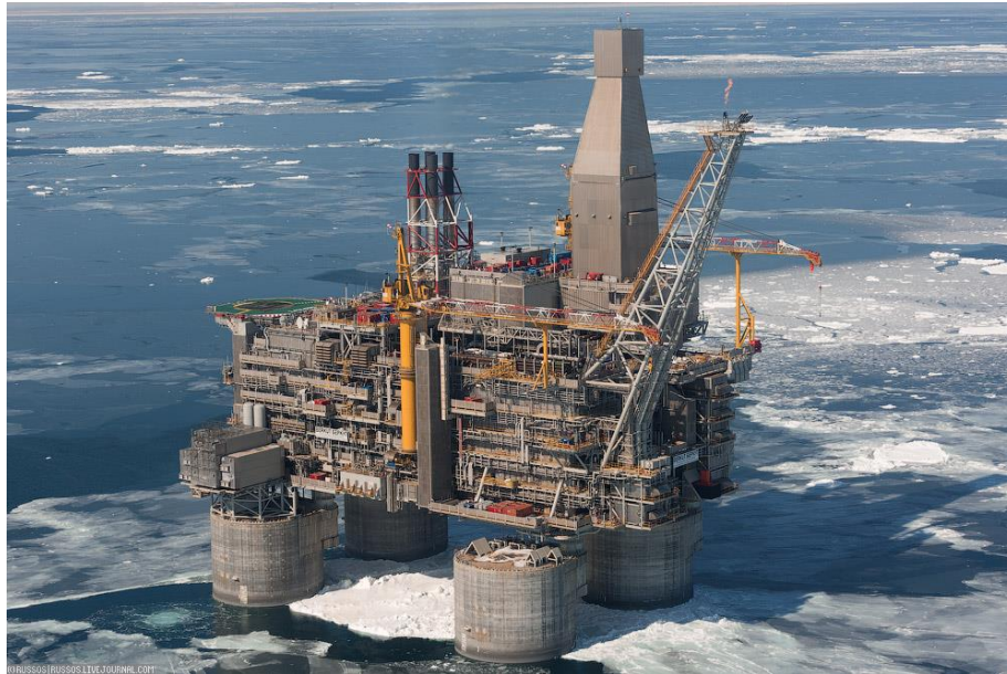
Figure 10. The «Berkut» platform (Photo courtesy of ExxonMobil Corp.)
