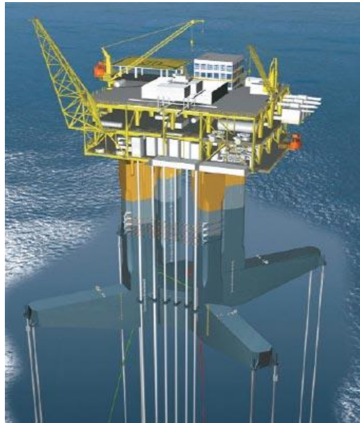
Figure 1-7 A Moses Tension Leg Platform (Offshore technology.com, 2016)
