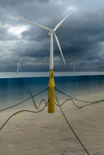
Figure 4-1: Illustrative picture of the Hywind concept, retrieved from [7].
